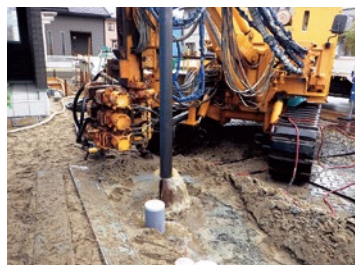
① 採熱孔掘削・鋼管建込
