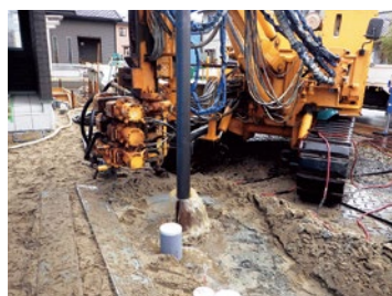
① 採熱孔掘削・鋼管建込
