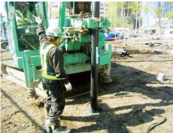
① 採熱孔掘削・鋼管建込
